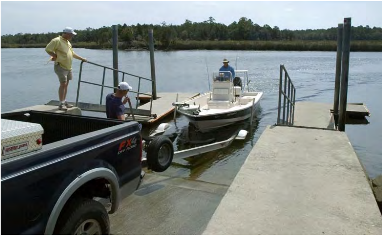
Florida has more than 200 freshwater boat ramps constructed by FWC using Federal Aid in Sportfish Restoration funds, credit: FWC
