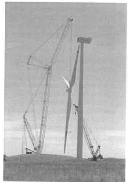
Towers are being lifted as work continues on the 2 MW Gamesa wind turbine that is being installed at the NWTC. Credit: NREL
