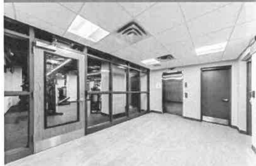
Figure 6.10 — It is important that there is a clear path of vision from the outside into the fitness room.
