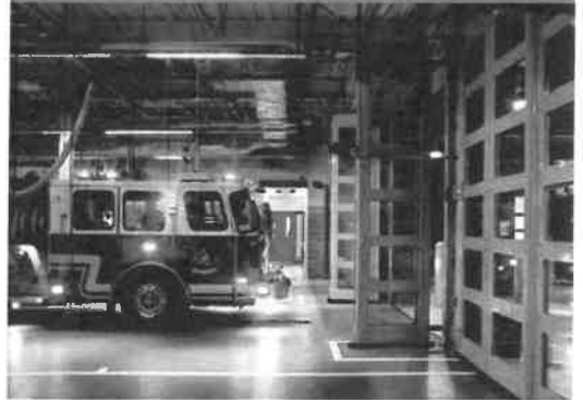
Figure 5.3 — A minimum 4-foot clearance shall be maintained (designed) around apparatus parked within the station.
