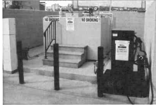
Figure 7.4b — These bollards protect the fuel pump and fuel storage.
