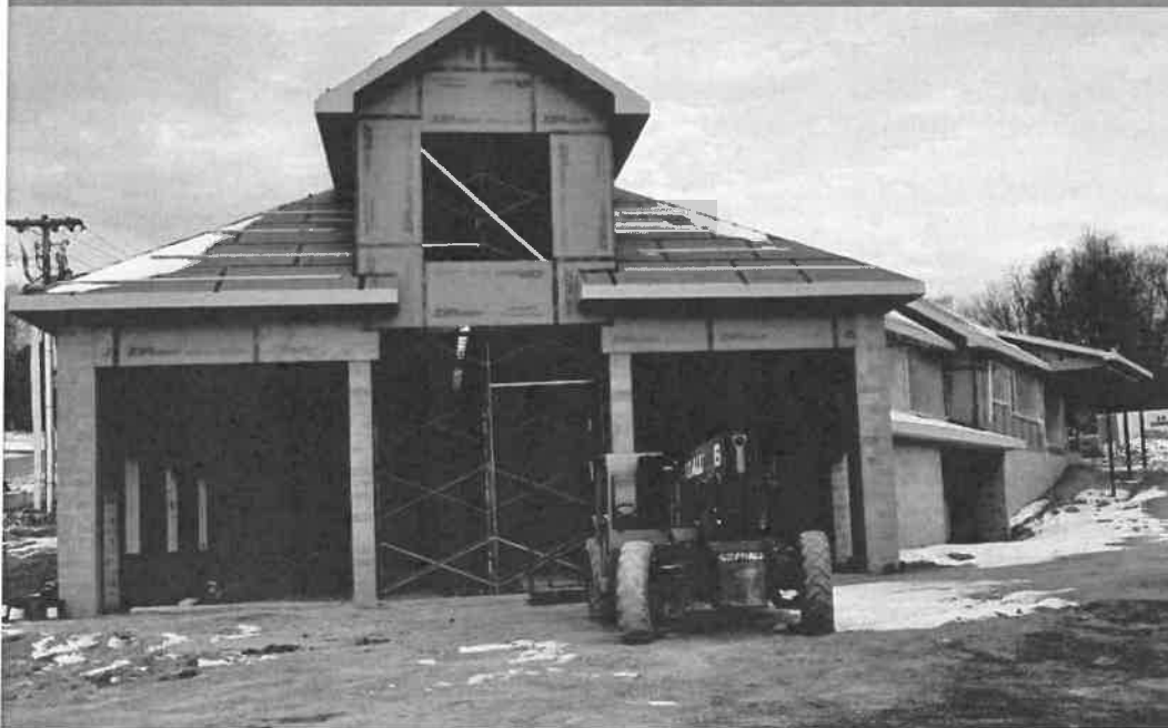
Figure 3.4 — This station being built on a hilltop is an example of a special construction consideration.
