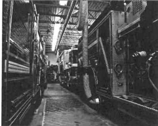
Figure 6.12 — A typical source capture exhaust filtration system.
