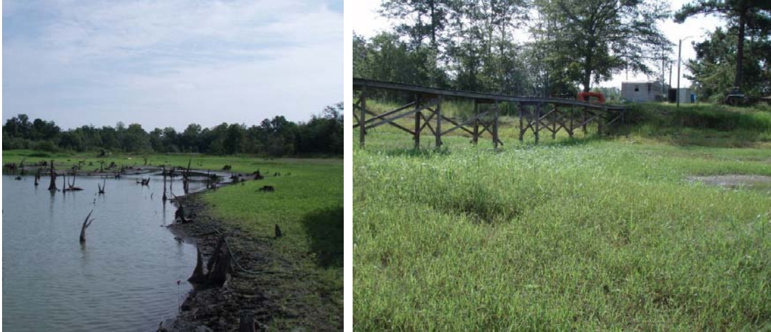
Figure 7. The water level is so low that there are no plants in the water and terrestrial plants are encroaching into the basin at a small pond.
